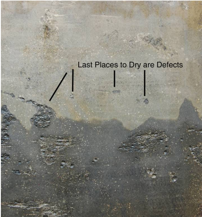
Figure 4 Field Drying and Concentration of Salts
